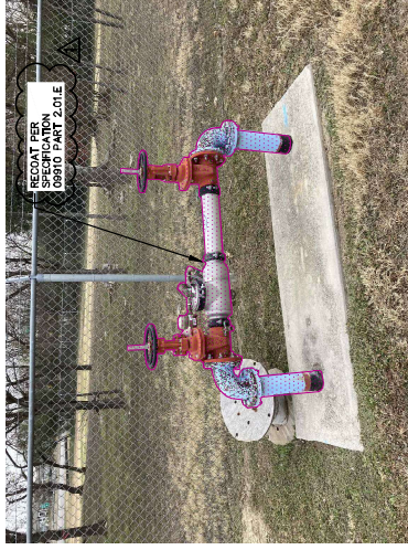
EXISTING ABOVE GROUND VALVE DETAIL
